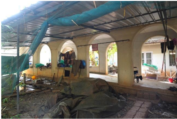
OUTDOOR AREAS CONVERTED TO EQUIPMENT DUMPING YARDS
